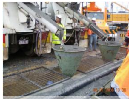
Tremie concrete placement
